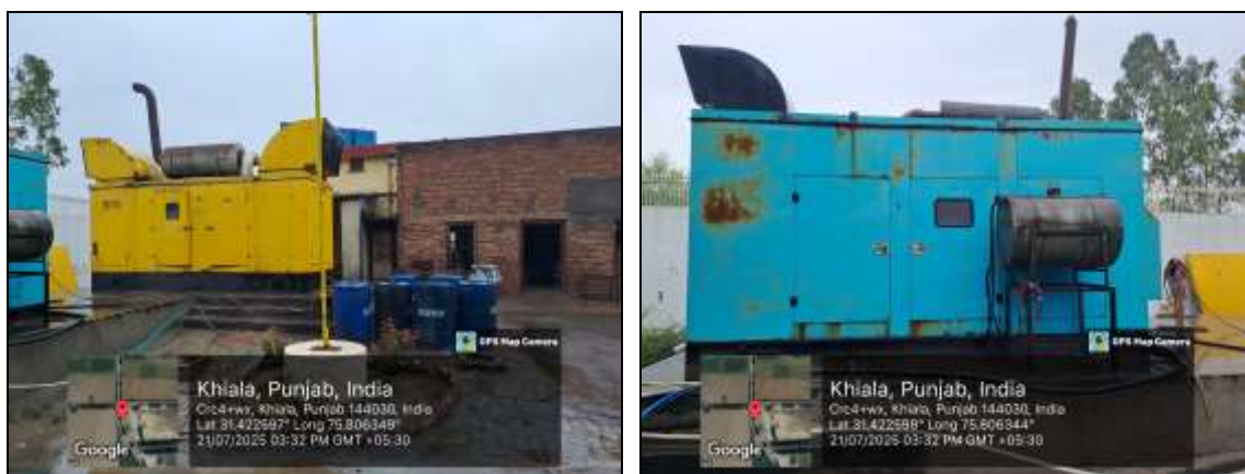
Existing DG Set 500 & 200 KVA installed in the university
